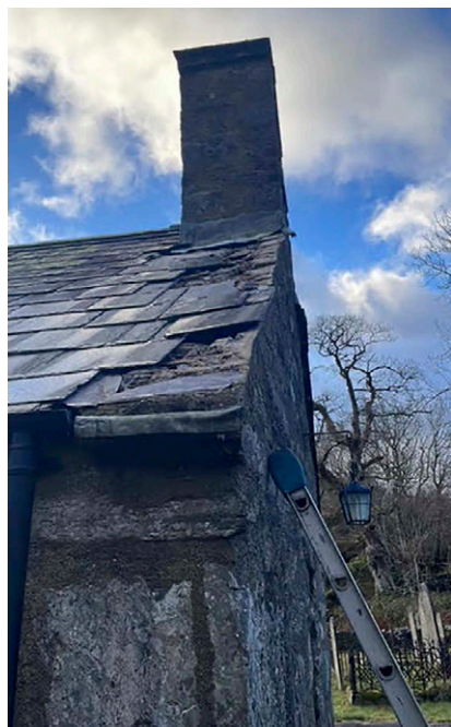
Slates blown off gable end of roof
